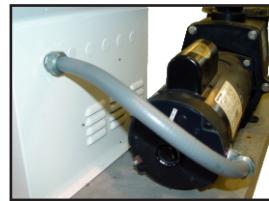
5) Route the other end of the conduit through the empty knock-out and secure with lock-nut. The cord inside will route up to the terminal strip inside the upper portion of the enclosure.
