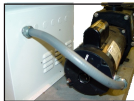
5) Route the other end of the conduit through an empty knock-out and secure with lock-nut. The cord inside will route up to the terminal strip inside the upper portion of the enclosure.
