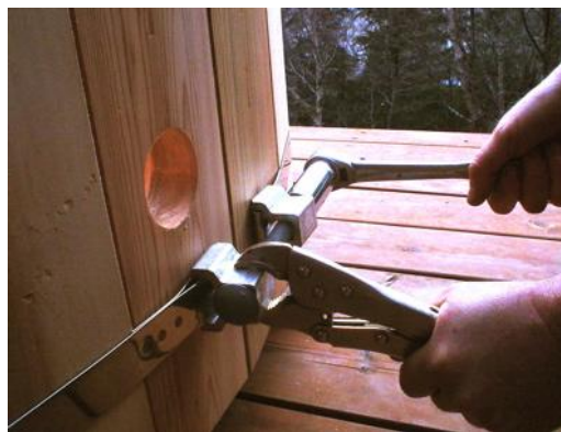
Figure 8.2 Using a wrench or pliers to hold the blocks straight as you tighten the bolt.
