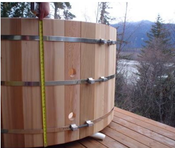
Figure 7.2 Proper placements of straps and bolts. Note how bolts straddle a seam between staves and are staggered.
