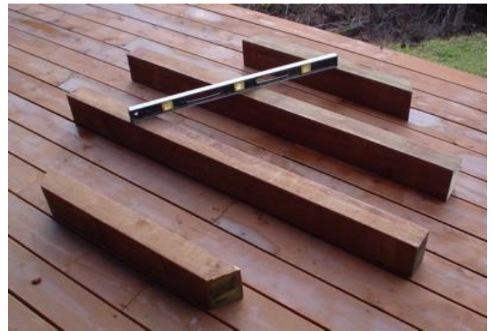
Figure 4.2 Level the chine joists
