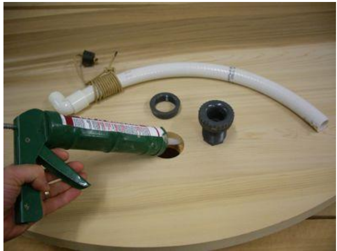
Figure 5.1 Drain assembly and silicone bead being applied to the recessed hole.
