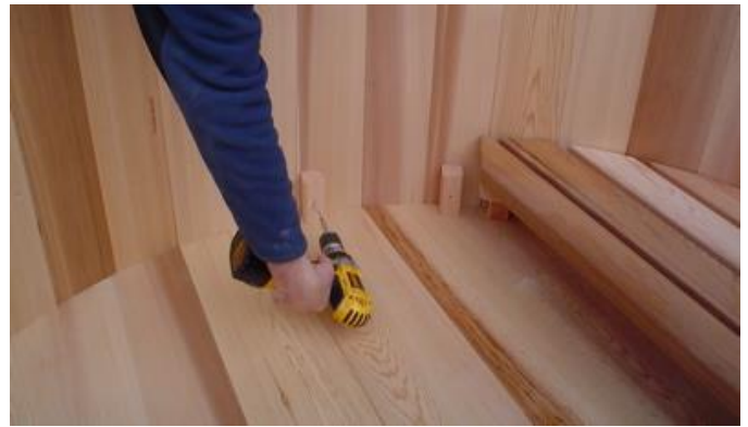
Figure 9.2 Aligning and attaching bench blocks – DO NOT drive a screw into a seam between staves! This will cause a leak.
