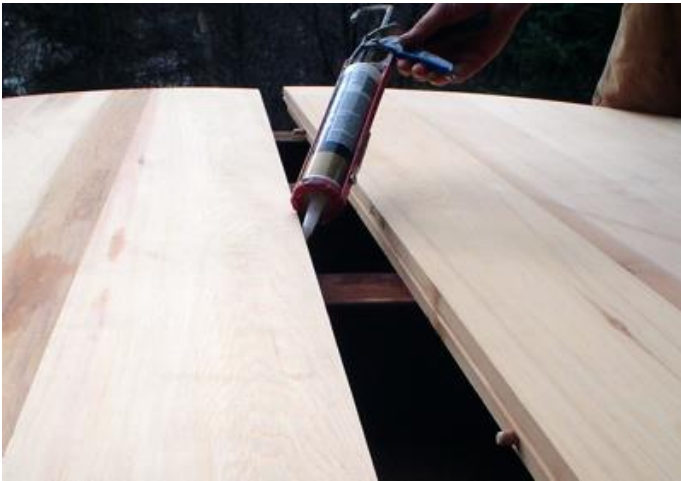
Figure 5.2 Floor seam, dowels and silicone
